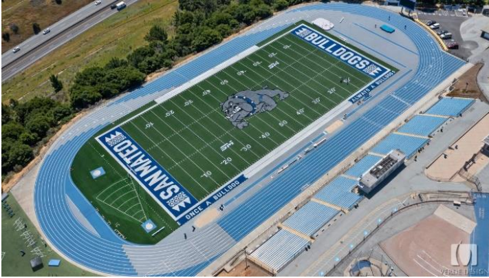
CSM Football Field and Track Replacement
